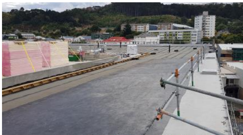
Roof vapour barrier complete to West and PIR & Poly stored on site
