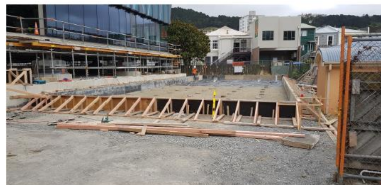
Services Annex Raft Formwork
